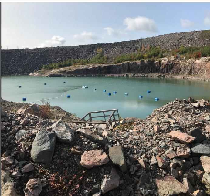
Barrels located in the Broken Hammer open pit are linked to the lime injection system, which is part of the process of treating effluent water before discharge.
